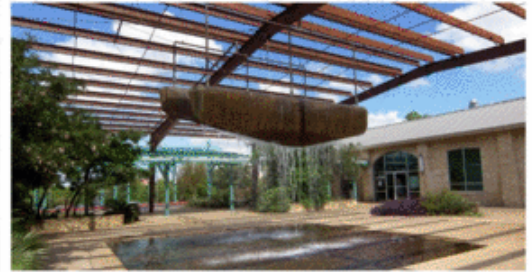
3601 South Congress- Existing Buildings
