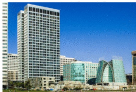
1 Kaiser Plaza – Existing Building
