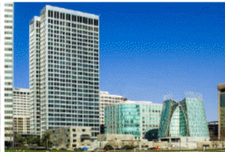
1 Kaiser Plaza – Existing Building
